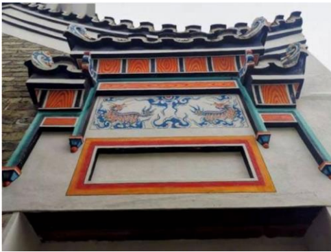
Figure 7: Xidi Village Paint at will.
