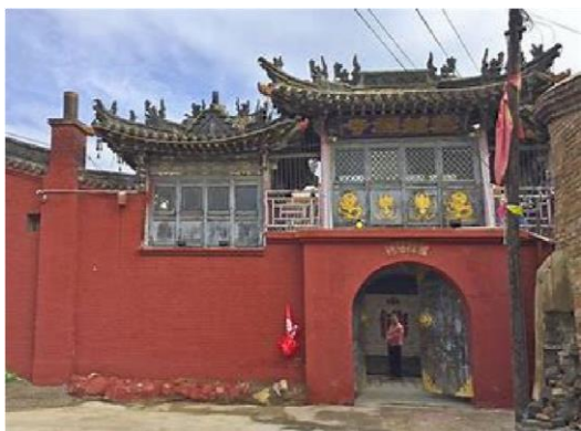
Figure 3: The situation around Datong ancient City Wall.
